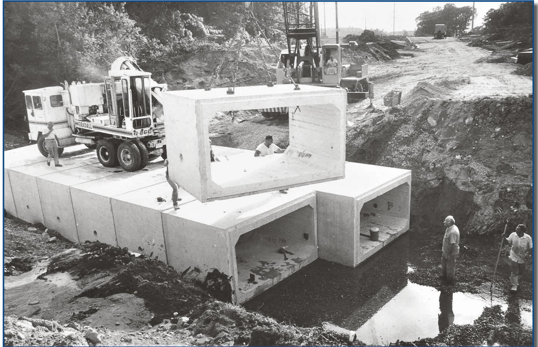
**Installing culvert on Flutie Pass, Natick MA, September 3, 1985**
