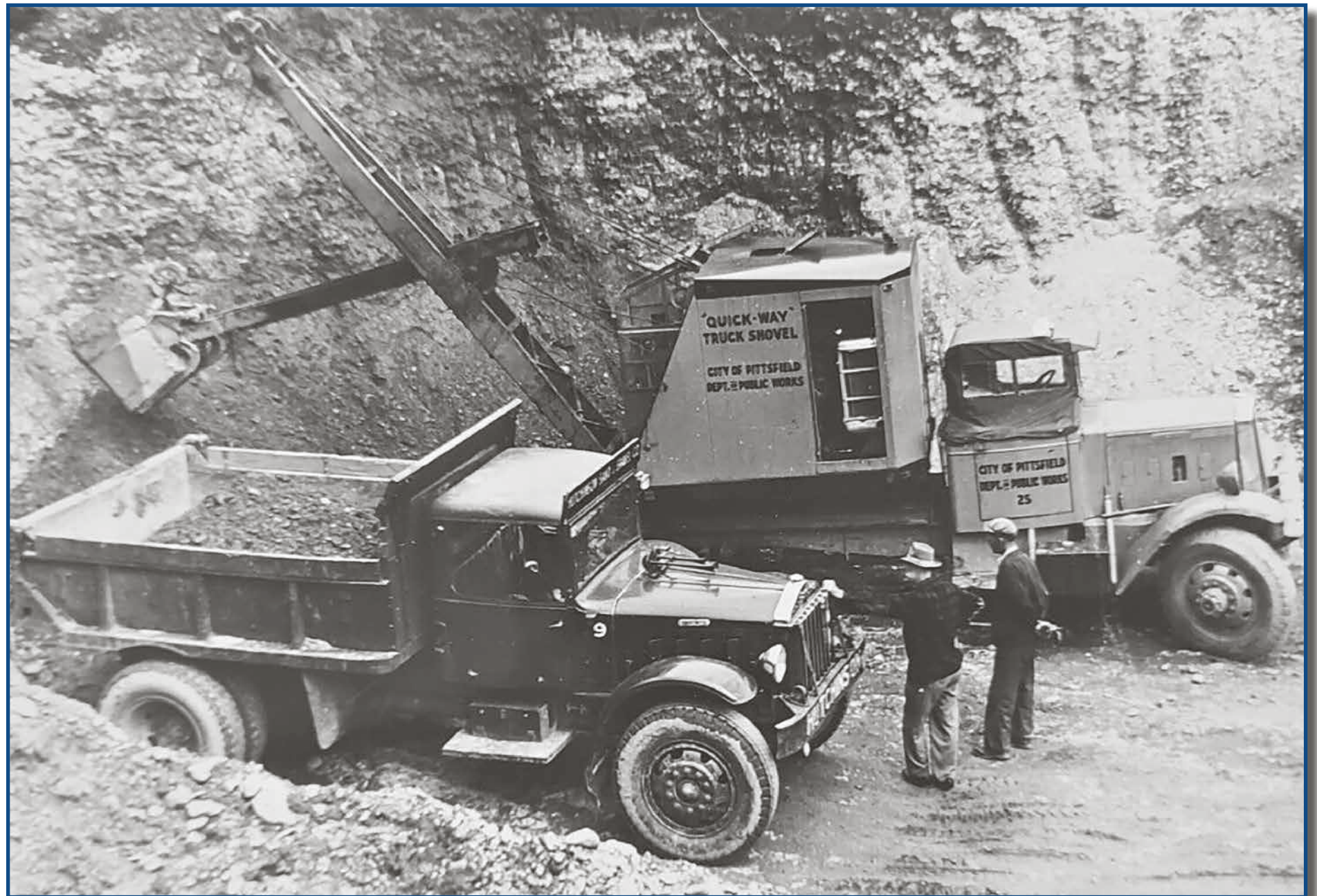
City of Pittsfield, Quick-Way truck shovel loading gravel into a Sterling dump truck, 1940s
