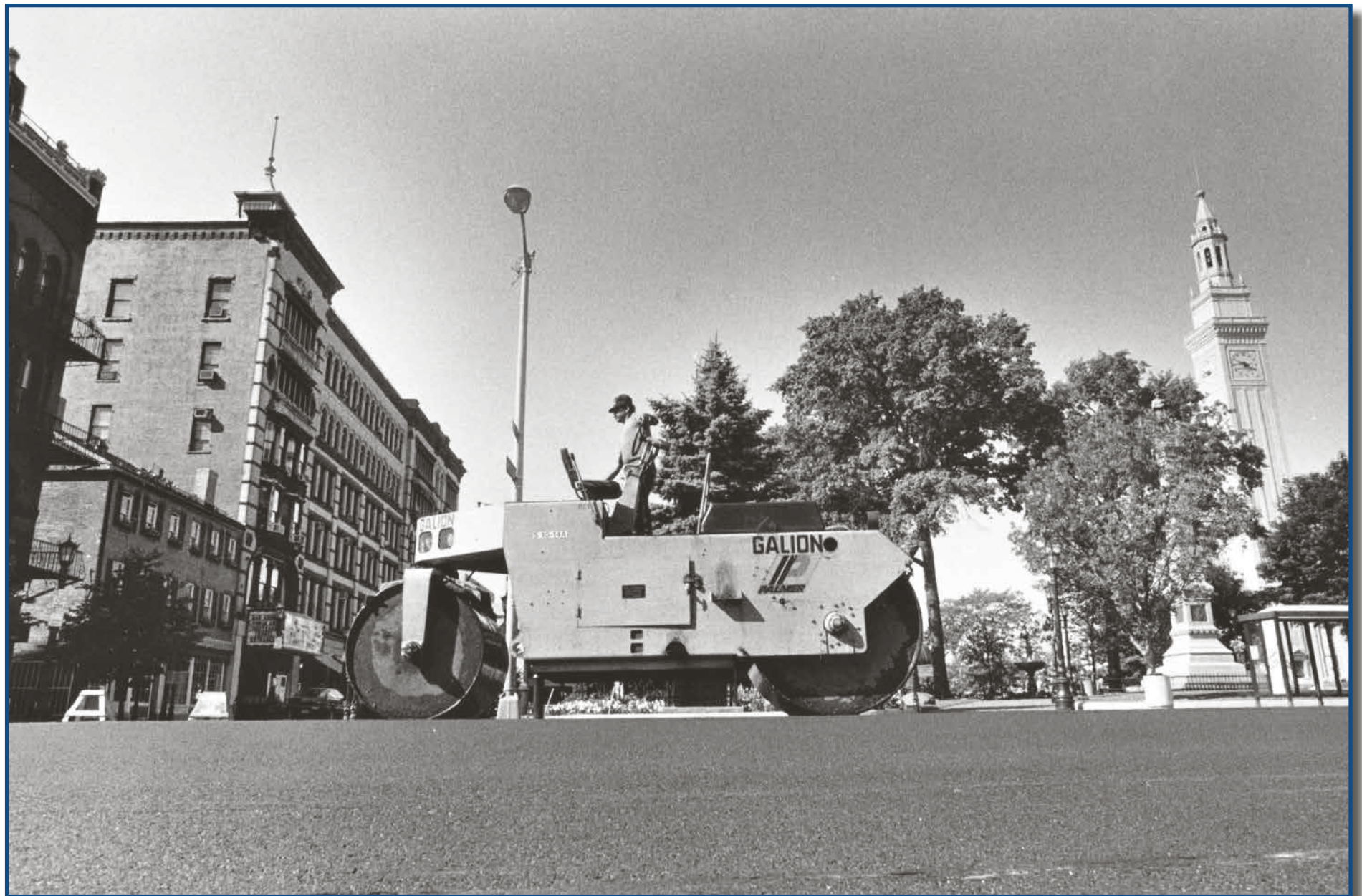
Galion roller compacting new asphalt on Main Street, Springfield, 1985
