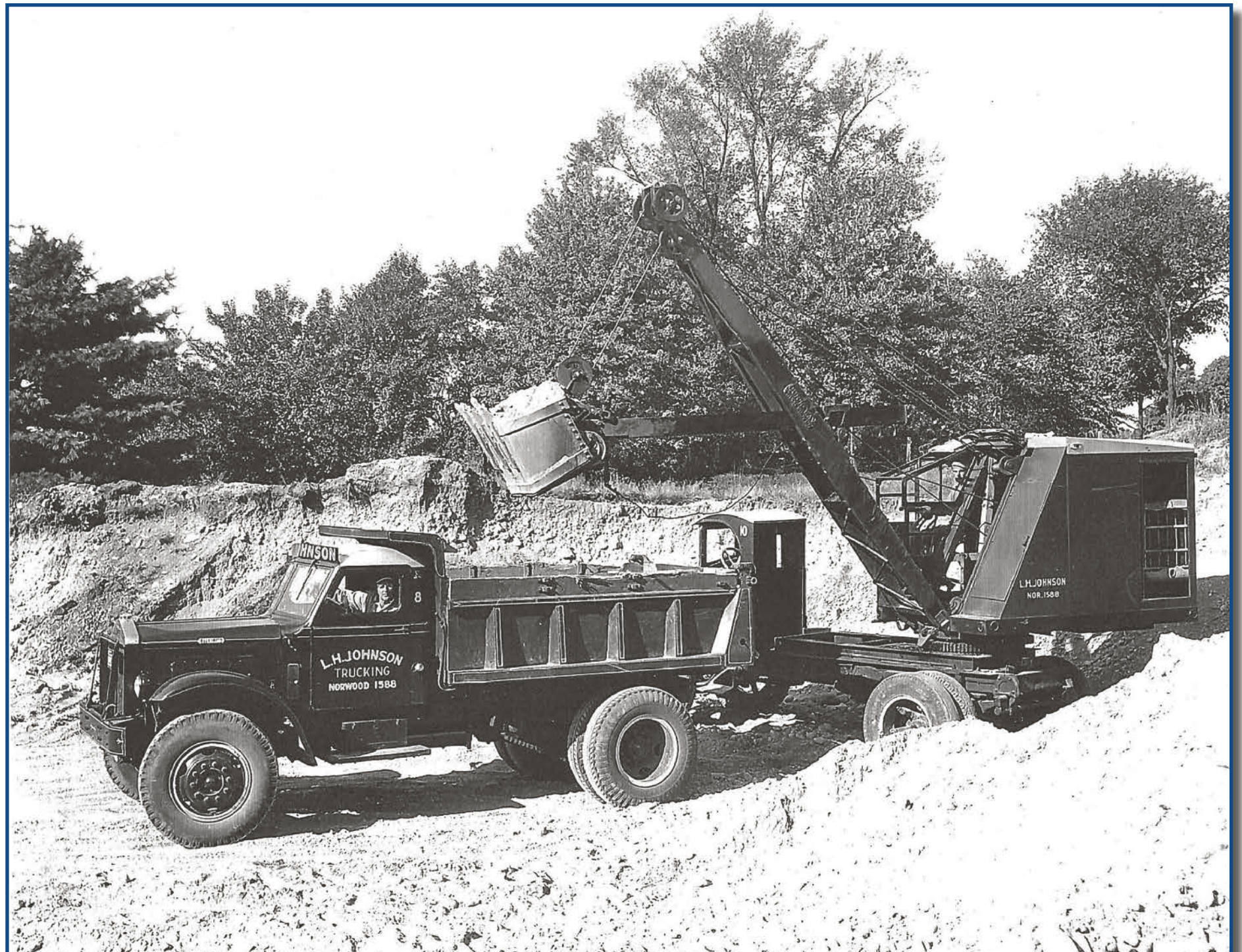
L.H. Johnson dump truck loaded by a truck-mounted Quick-way shovel, 1940s
