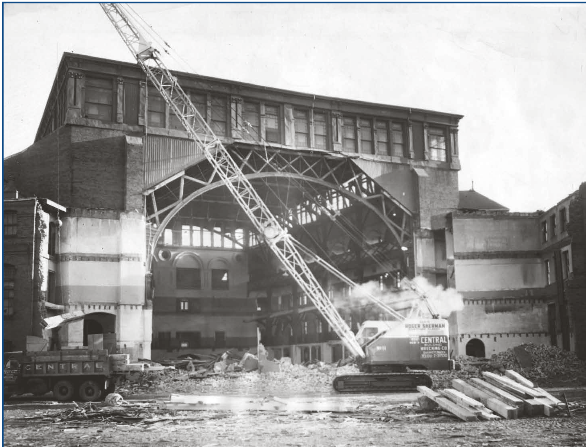
Roger Sherman crane demolishes Mechanics Building in Boston, 1958
