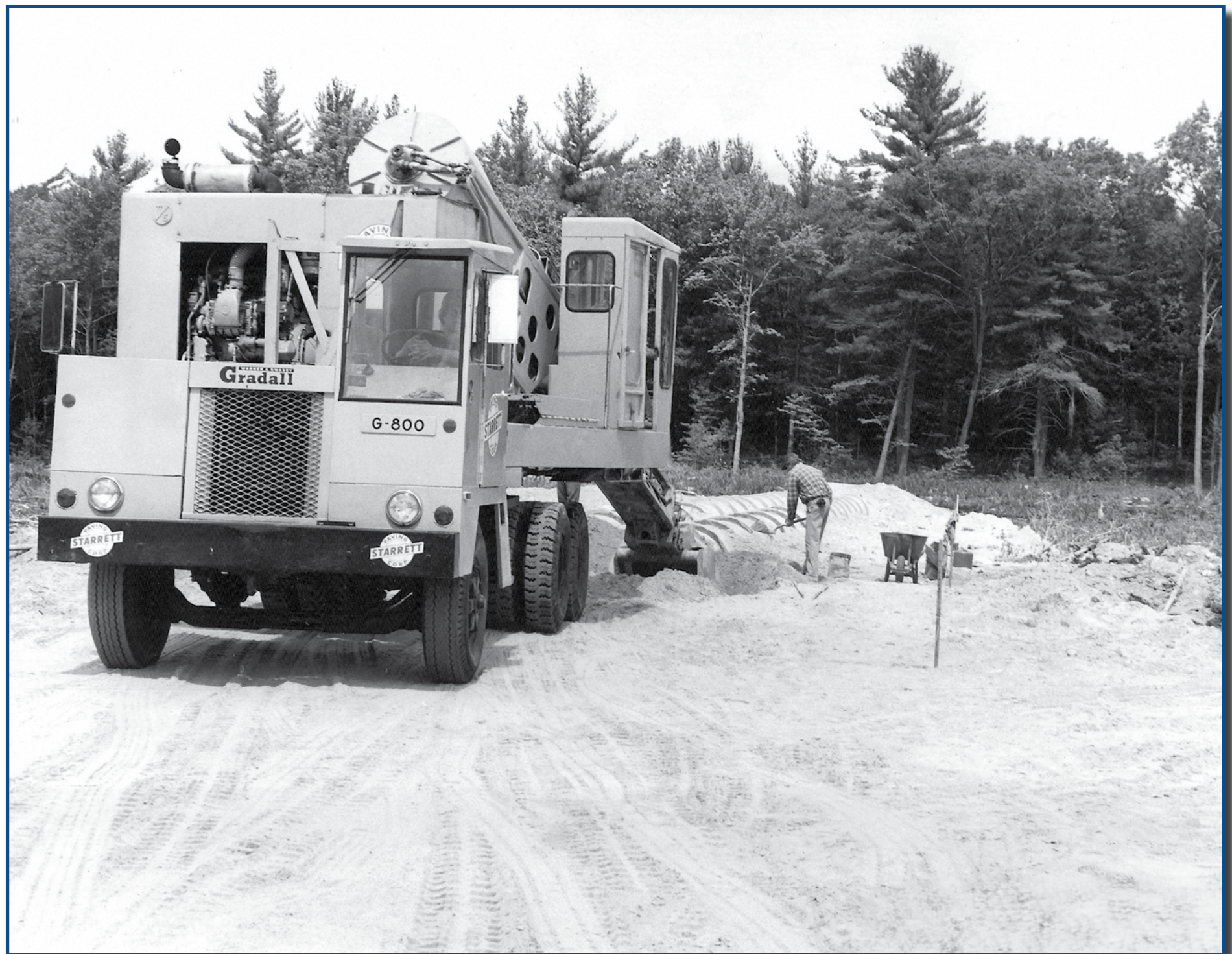
Starrett Paving Company, Gradall installing twin 36-inch concrete drain pipes on Interstate I-190 in West Boylston - Holden for M. DeMatteo Construction Company. 1980
