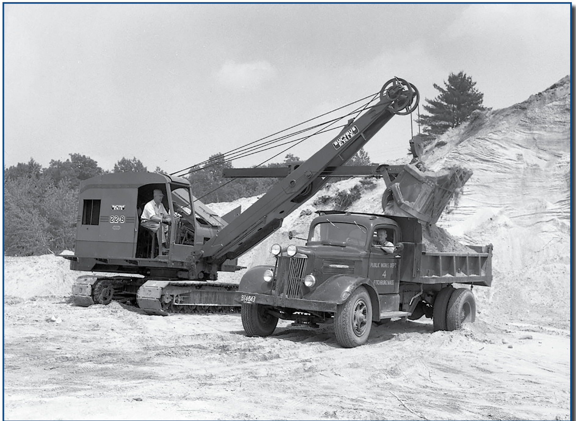
Fitchburgh Public Works Department loading White dump truck with Bucyrus-Erie shovel 1950s.
